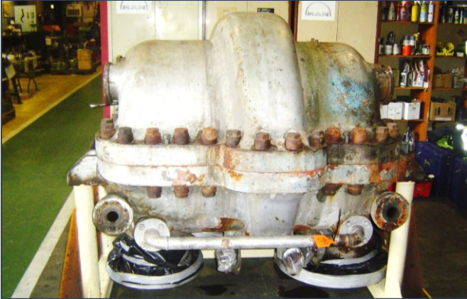
Ammonia syngas turbo compressor overhaul at the workshop
