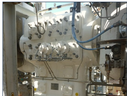
Onsite overhaul of natural gas, oxygen, CO 2 , hydrogen compressors
